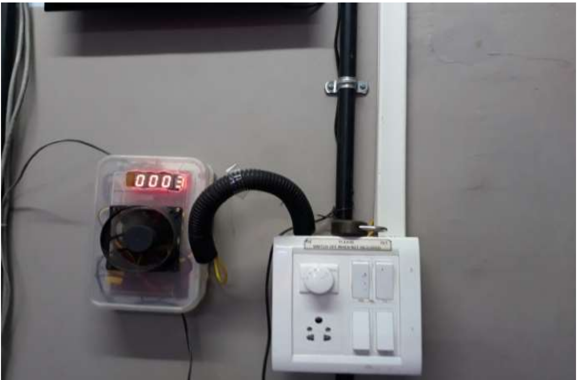
Image 3 – Room automation console
